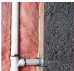
Cellulose insulation on the right Fibreglas insulation on the left
